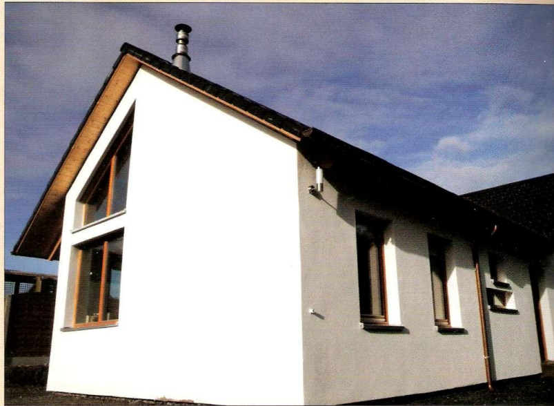
(above)The Malahide house is a mixture of timber frame and timber dovetail construction and was completed within just two months of the start date; (next page top) sun light illuminates the timber of the roof overhang; (next page bottom) The couple, Pam O'Donnell and Marcel Laskody, at home in their new house
