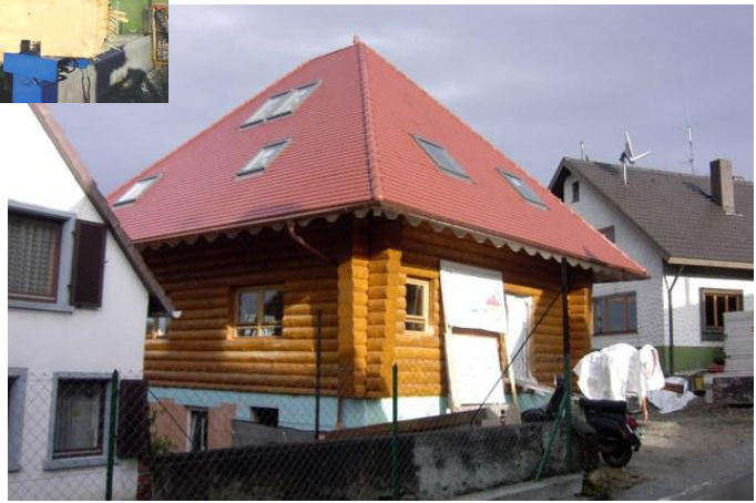
1-layer Log Cabin System, Primary Energy Need: 48kwh/m2/Jahr – WITHOUT any extra insulation!
