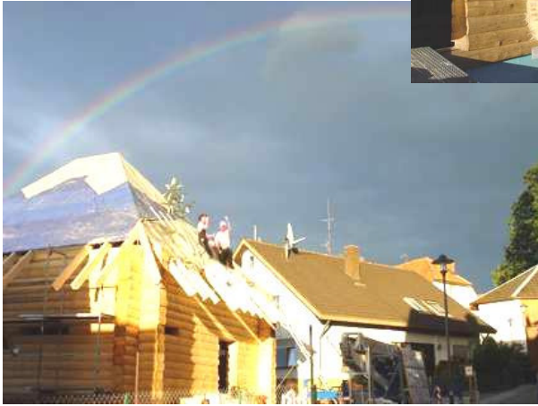
1-layer Log Cabin System, Primary Energy Need: 48kwh/m2/Jahr – WITHOUT any extra insulation!
