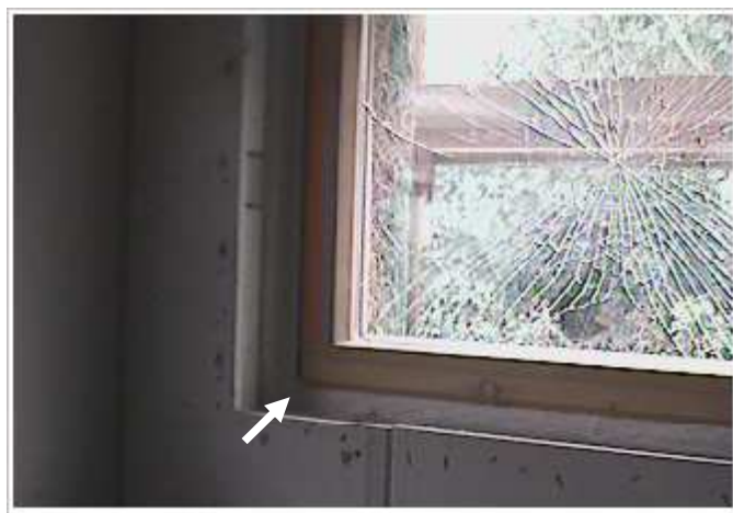
Figure 22 East Windows North Corner – Visible
