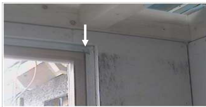
Figure 5 West Window – Visible
