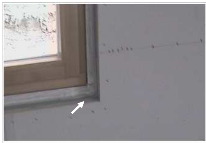
Figure 14 East window right hand side - Visible
